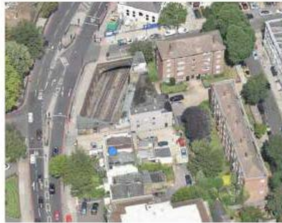
View of railway cutting (top) and aerial view of site looking south (bottom left) and aerial view of site looking north (bottom right).
